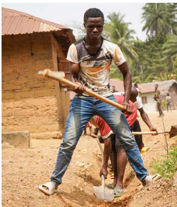
Community digging ditches to divert rainwater
