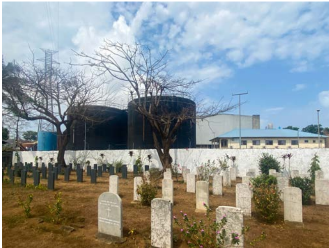
(a) Kingtom Power Station
