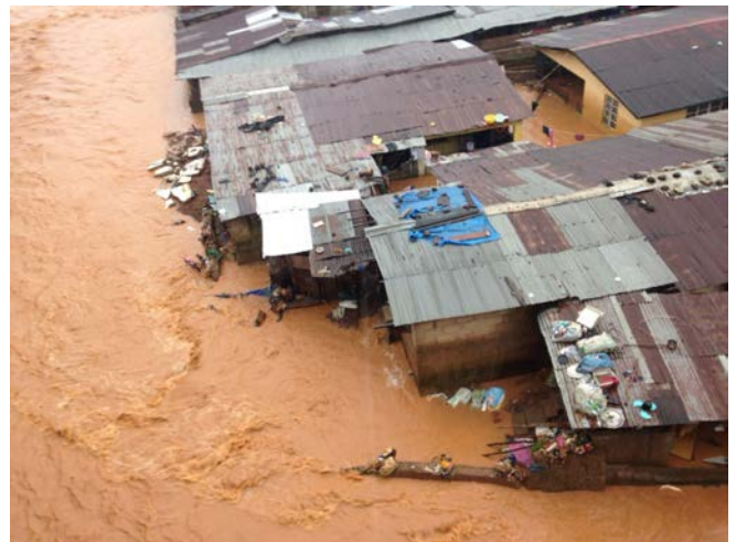
Figure 4: Flooding in Freetown
