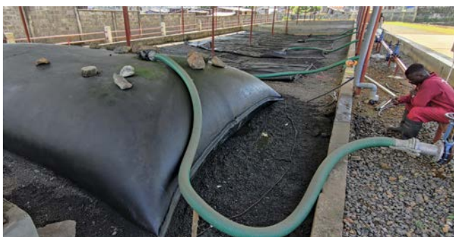
Figure 28: Geo-tube dewatering system
