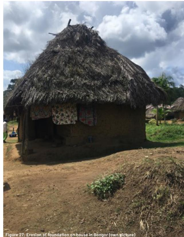
Figure 27: Erosion of foundation on house in Bongor (own picture)
