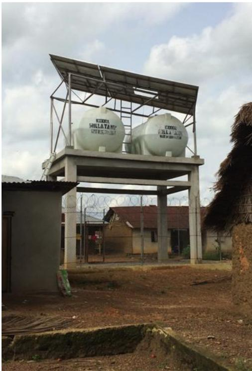
*The water tower is designed to contain 20 m<sup>3</sup> of water. The construction is a concrete scaffolding.*
