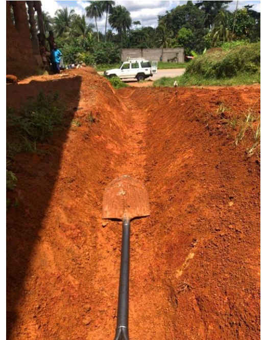
Figure 1 – 30, 20, 10inch drain with shovel blade (10inch) for the drain's bottom measurement. Talia
